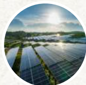
Solar panel fields
